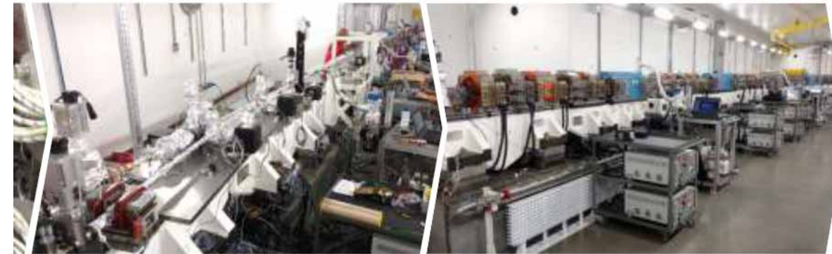
An Overview for the Sirius Vacuum System, T. Rocha, EIC 2021
